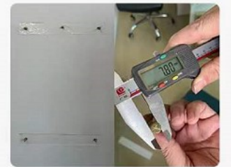
6 drill hole,insert the screw
